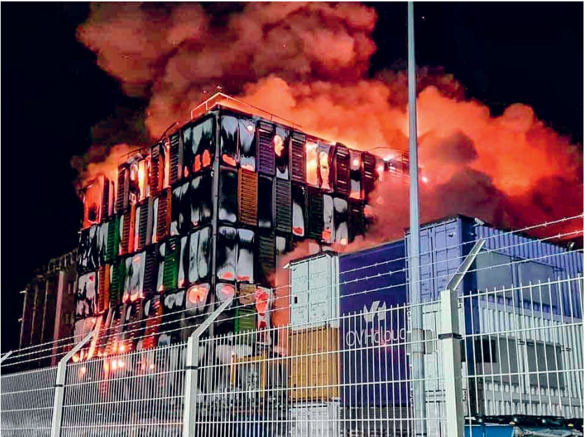
Major fire at the data center cluster OHV in Strasbourg, France, on March 10, 2021
