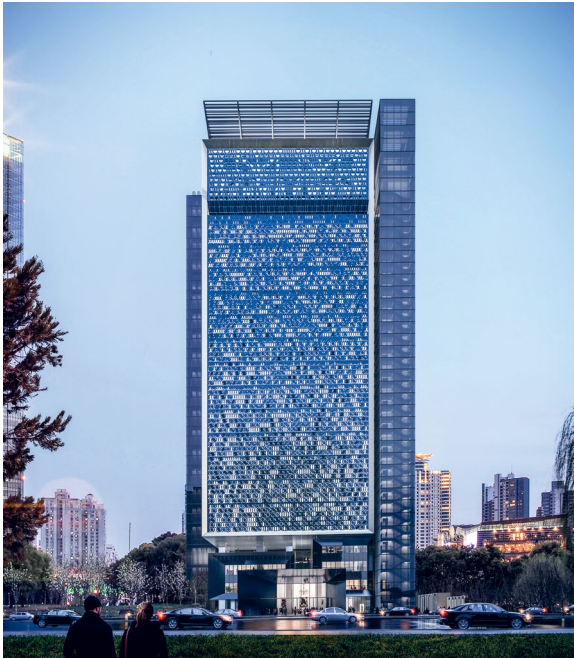
Qianhai Telecommunication Center, Shenzhen, China
