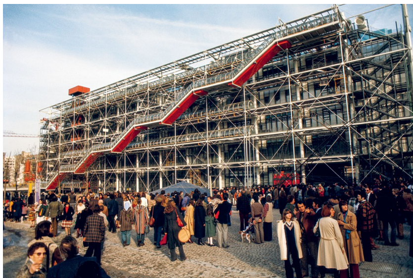
Centre Pompidou, Paris, France, 1977
