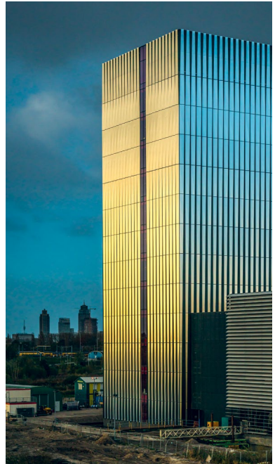
Equinix AM4 data center, Amsterdam, Netherlands
