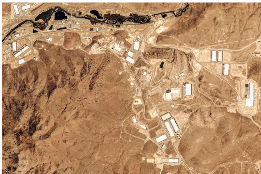
Tahoe Reno Industrial Center (TRIC), Nevada, USA
